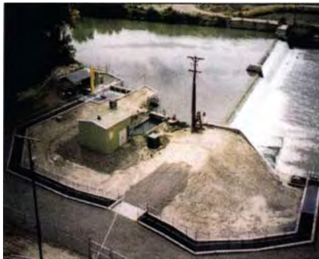
(b) Fish passage facility at Redlands Diversion Dam on Gunnison River, Colorado.
