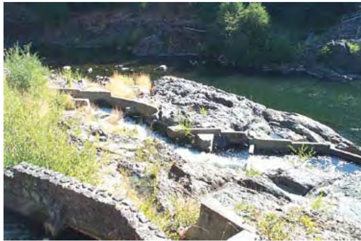
(a) Vertical slot Potter Valley fish ladder on the Eel River in California.
